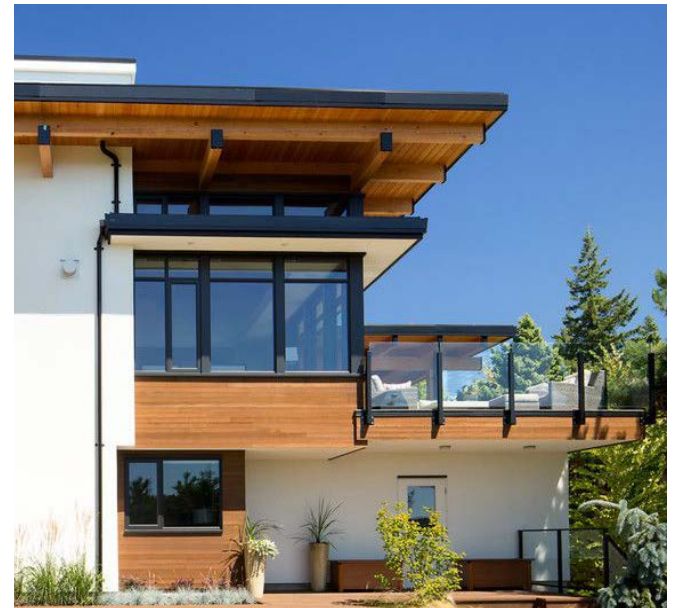
Exposed beams with modern downspouts & metal trim.
