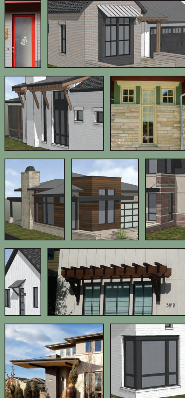
Elements such as dormers, gable ends, covered entries, building projections, window packages, and color help break up long expanses of blank wall areas
