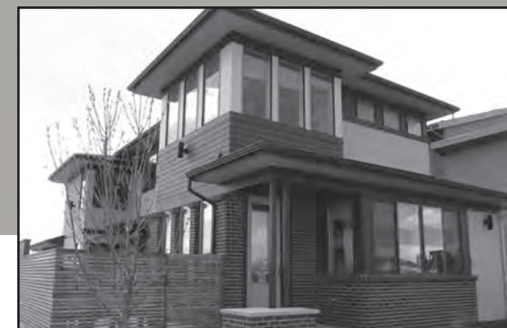
Traditional low-pitched hipped roof, low-pitched porch covering, and an example of a style specific door.
