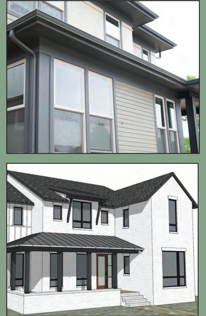
Deep roof overhangs create depth, shade, and shadow, reflecting the architectural style of the home.
