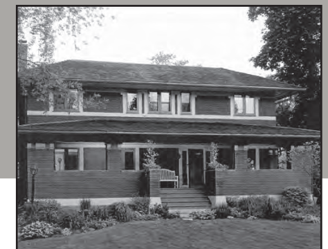
Ribbon windows hug the eave line and are accented with horizontal siding that clearly establish a horizontal image.
