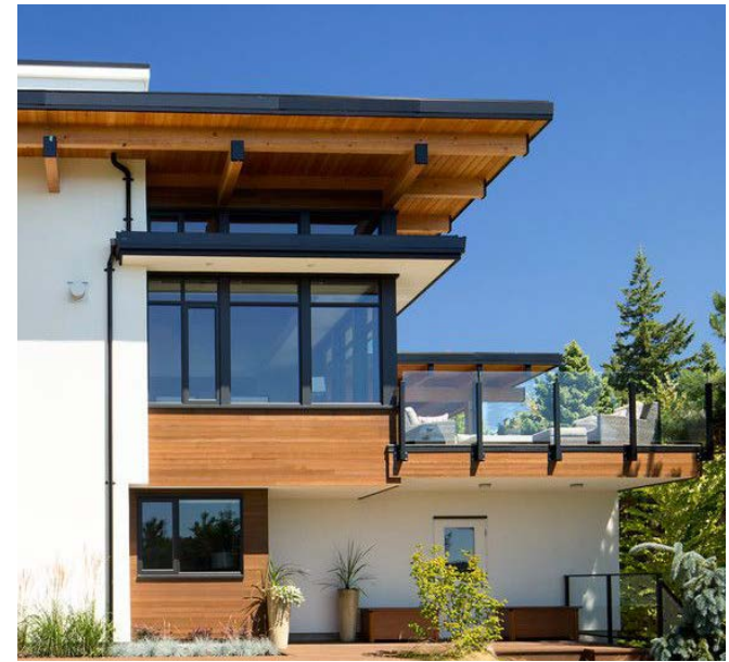
Exposed beams with modern downspouts & metal trim.
